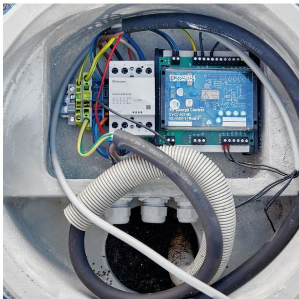
Charging controller according to IEC 61851 Mode 3
