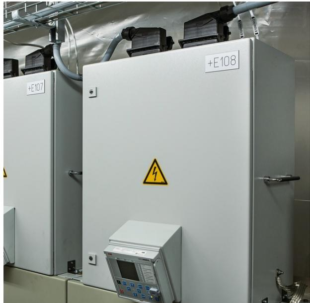
HEAVYCON EVO connector for connection at the control cabinet
