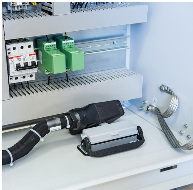
The locking latch makes the connection easier and more secure
