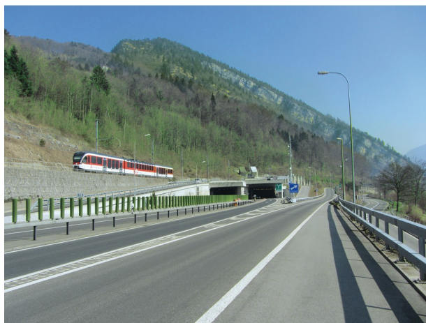
Lopper Tunnel in Switzerland
