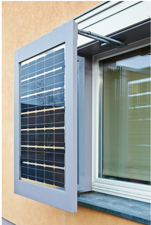
The PV shutters can be tilted in parallel to the window
