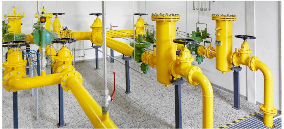
*In addition to monitoring the gas pressure control (8 bar to 50 mbar low pressure) the supply quantity, for example, is now detected via the Ethernet extenders.*
