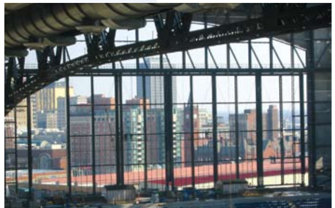
A view of the kinetic wall inside the stadium during construction
