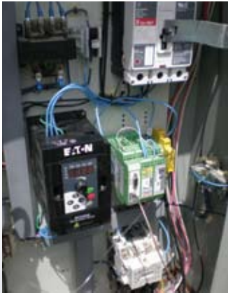
Phoenix Contact Trusted Wireless data radios monitor and report on the mine's pumps and flow meters.
