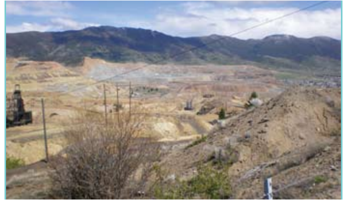
Because of the difficult terrain and remote nature of the wells, traditional monitoring systems could not be used.
